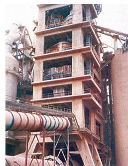
Figure 33. This is a lime kiln which decomposes calcium carbonate (limestone) into calcium oxide (or lime).
