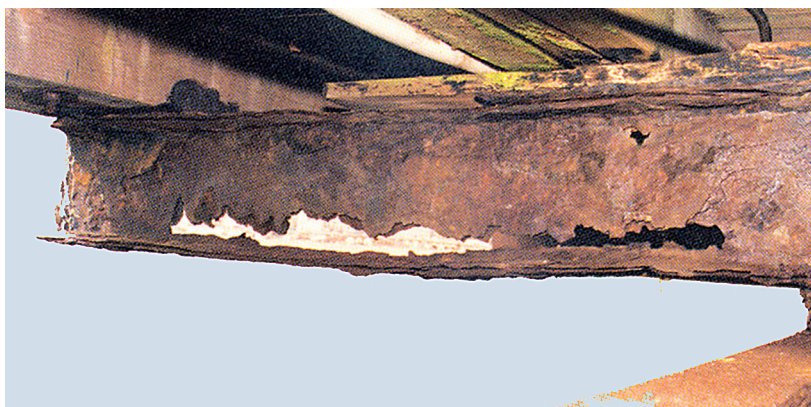
Figure 56. This picture shows the eating up of an iron object due to corrosion (or rusting) caused mainly by the oxidation of iron by oxygen of air.
