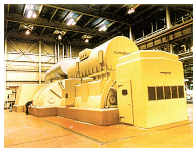
(a) This is a very large power house generator. It produces alternating current (a.c.)
