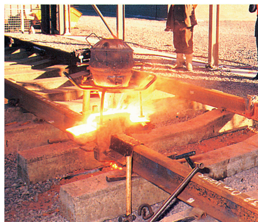
Figure 78. This picture shows thermite welding of broken rail track. The molten iron formed from the reaction between \text{Fe}_2\text{O}_3 and \text{Al} is run into a mould around the rails to be welded (or joined). When the molten iron has cooled, the mould is removed, and excess iron trimmed off.
