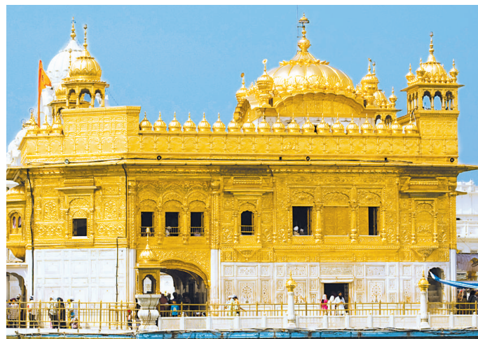
Figure 92. Gold metal is used in leaf form on 'Golden Temple' as it is highly unreactive and does not corrode on exposure to air. The thin gold leaf coating not only adds long-lasting beauty, it also protects the marble structure beneath from corrosion.
