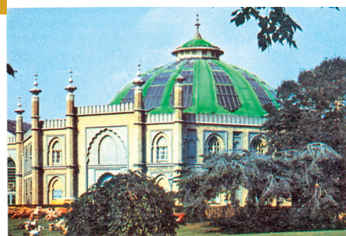
Figure 90. Copper metal corrodes in air to form a green substance called basic copper carbonate. The copper dome over this building is green because copper metal has reacted slowly with the carbon dioxide and moisture (water) of air to form a green coating of basic copper carbonate.
