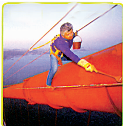
(a) The iron pipe is being painted to prevent rusting
