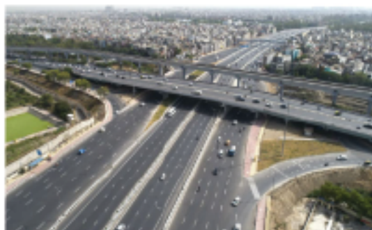
Kundli Manesar Expressway
